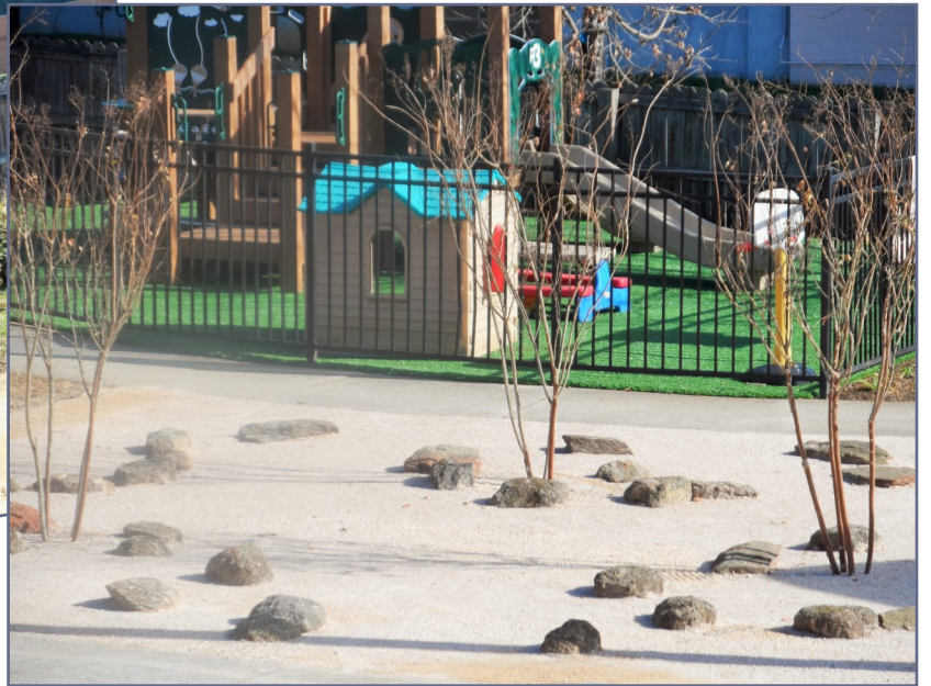
The Outdoor Learning Classroom Under Construction
